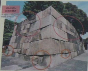
崩壊部、隙間 Damaged or separated masonry
